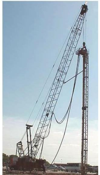
The installation sequence consists of using a long crane-mounted auger rotated down to full penetration, then pulling out the auger (while continuing the rotation) and while pulling, pumping the concrete down the center shaft of the auger to fill the hole from the bottom up. After extraction of the auger, the rebar cage is dropped or vibrated in. The concreting and reinforcing operation must take place in 45 minutes to ensure no early setup.
