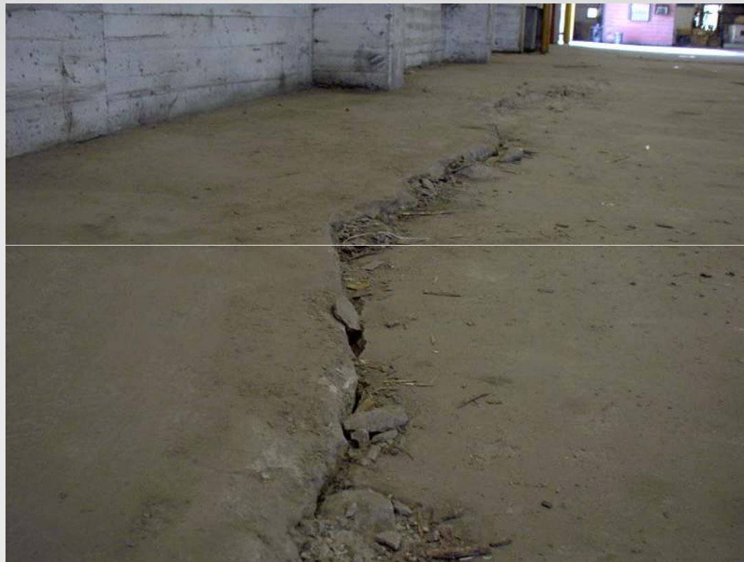
Slab failure near exterior grade beam due a large void.
