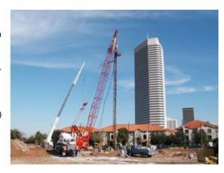
Mr. Brettman said his company also installs APG piles that are partial or full Displacement (called APGD), for use in loose or soft soils. The drill string consists of a short auger with a solid collar above and a smooth and smaller-diameter drill stem to the surface. The collar displaces the soil cuttings laterally to help keep the hole open. A special drill rig from Europe is needed to install AGPD piles that has several times the torque than the crawler cranes used for AGP piles provides.
