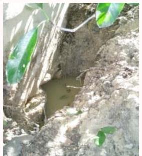
Water ponding at grade beam / pier
