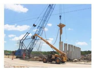
Mr. Boehm said his company has installed over a hundred miles of 3 to 4 ft diameter stone columns penetrating 10 to 55 ft in the Houston area using limestone rocks up to 3" in size. They tend to pre-drill the hole if it will stay open, and if not, they will vibrate a hole and drop the rock around the annulus. They also can force the stone via air pressure to the bottom and vibrate as they pull out of the hole. They usually have to keep at least 25 ft away from existing buildings when vibrating.
