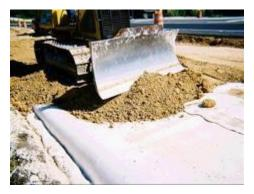
course with a slope toward the pavement edge where a French drainage type system is installed to move the water away from the pavement.
