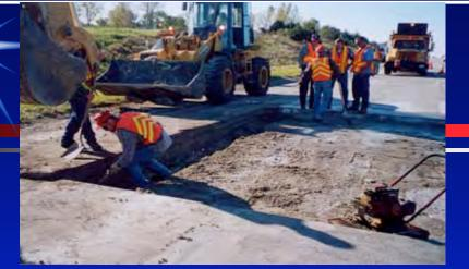
A drainage trench must be dug at the edge of the road to collect moisture that drains through the JointDrain.
