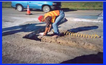
Applying epoxy into dowel holes before placement of dowel rods
