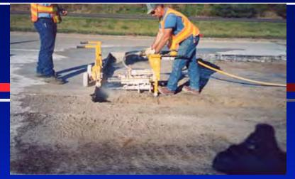
Drilling dowel holes at the edge of each concrete "cut"
