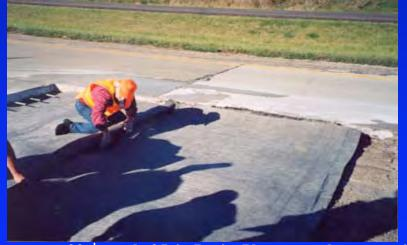
Placement of 2<sup>nd</sup> panel of JointDrain. Please note that geotextile is shingled from 1 panel to the other where the panels meet. This keeps drainage course free from concrete debris.
