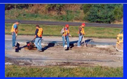
**Clearing debris to prepare subgrade**
