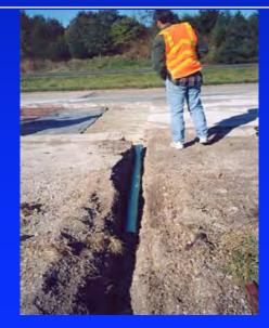
A Perforated PVC Pipe is placed as a drainage outlet at the end of the 25' section.
