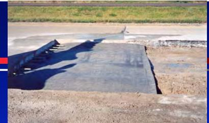
Placement of 1<sup>st</sup> panel of JointDrain. The panel is installed under the dowel bars with the main drainage path going towar the drainage trench.
