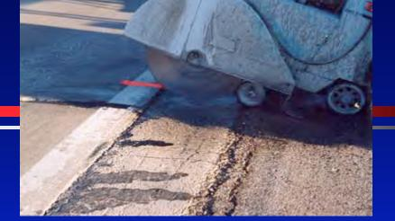
Cutting out a 25' section of concrete between 2 failed concrete joints
