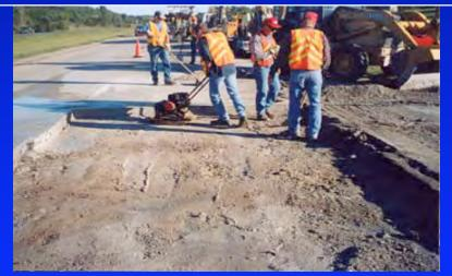
Compacting subgrade in preparation for the installation of JointDrain
