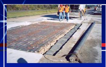
After last panel of JointDrain is placed, metal mesh is placed. Metal mesh is rested on dow bars, and on top of JointDrain panel.
