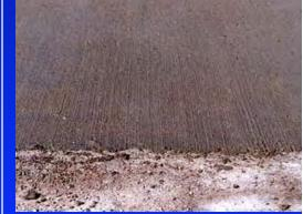
The final poured concrete that poured on top of JointDrain order to repair 2 faulty concre joints.
