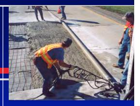
Screed is used to smooth and fla the poured concrete.
