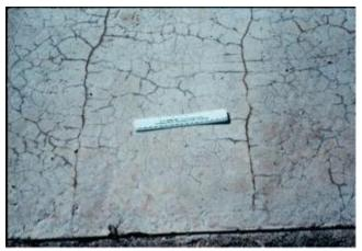
layer. An old rule of thumb for the evaporation rate of concrete was 0.2 lbs. water/SF/Hour, however it can be less now depending on the additives used in the mix. Factors causing rapid moisture loss include concrete and air temperature, relative humidity, and wind velocity. Plastic shrinkage cracks are normally shallow, short, and parallel.
