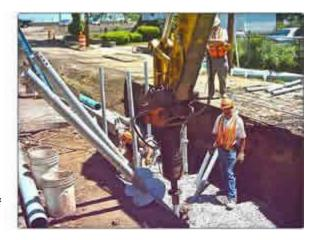
The information presented by Mr. Deardorff indicates that helical anchors and piles are a versatile foundation system for compression and tension loading applications. They primarily work in axial loading and take advantage of the bearing capacity of helical screw plates (helix) located along either round or square steel shafts. Fundamental steps to design with helical anchors and piles were presented along with installation and load testing protocol.
