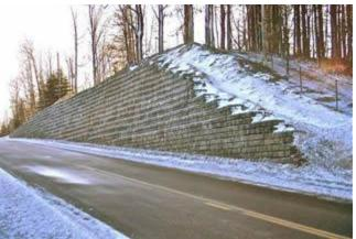
with a keyway slot on the bottom of the next course. The interconnecting geometry allows aesthetic curves along the wall. The standard block size measures 18" high by 46" along the face of the wall by 41" deep.
