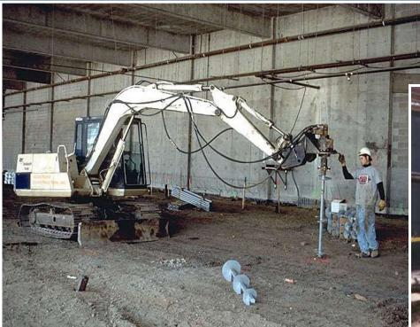
Helical Piles Supporting Structural Slab
