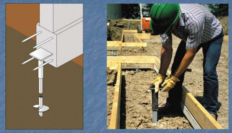
C150 0458 for 1  $\frac{1}{2}$ " Square Shaft 40,000 lb design load C150 0459 for 1  $\frac{3}{4}$ " Square Shaft 60,000 lb design load
