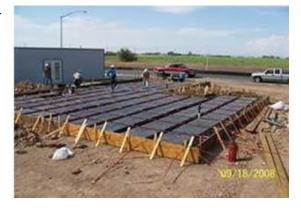
through the footprint and perimeter. The system can be installed easily by a local concrete provider and offers building cycle time reduction and cost savings by eliminating trenching time, moisture barrier installation, pad presoaking, and reinforcing supports. Variable height, fold-out tendon supports are included in the original molding process so there are no loose pieces to install.
