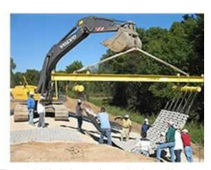
blocks are also designed allow for expansion and contraction. The special block shapes also provide for additional interlocking restraint. The systems may be hand placed or installed by crane as large pre-assembled mattresses. Some of the key points presented were:
