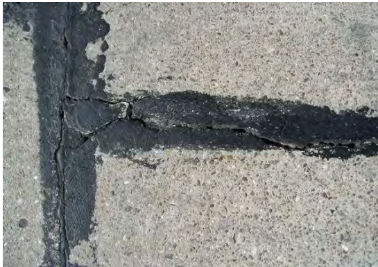
Joint & crack sealant deterioration
