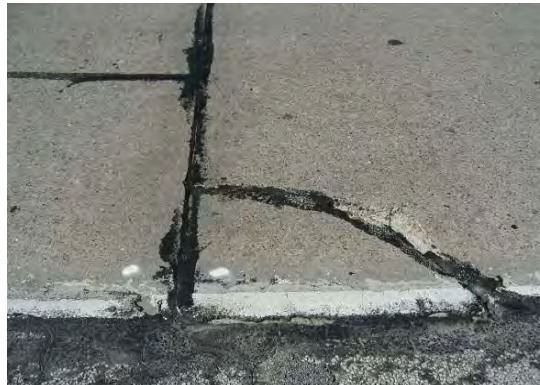
Joint & crack sealant deterioration
