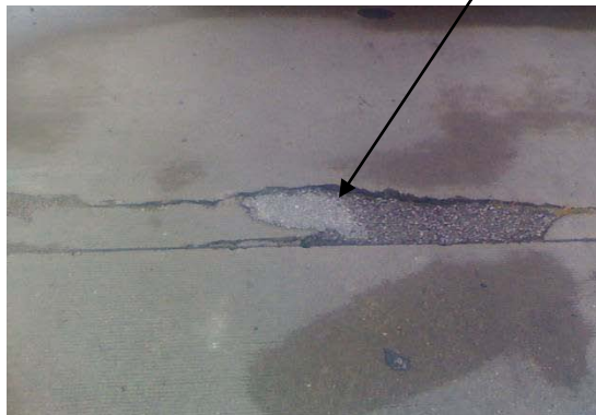
Transverse cracks near joint
