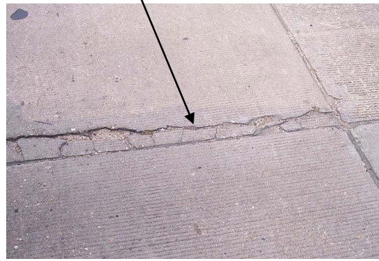
Transverse cracks near joint
