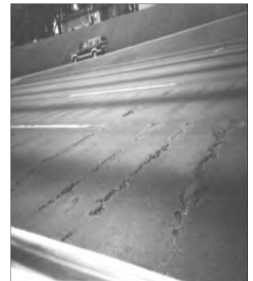
Figure 1-1 Spalling in concrete pavements [Soares and Zollinger 1998].
