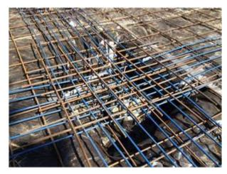
The post tension slabs are typically designed as two-way slabs without drape considerations. The slabs are supported on a grid of piers with an average pier spacing of twelve to fifteen feet on center. Slab thickness is typically in the six-to-seven-inch range. Thickened areas with rebar are typically used around supports or regions of high shear. Grade beams are not required although a perimeter beam is typically employed for moisture control.
