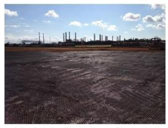
Tensar has long been an innovator in offering cost saving solutions for both traditional and non-traditional applications. Keith stated that millions of dollars have been saved on laydown yards, heavy haul roads, crane pads, and rail lines by utilizing Tensar geogrids on these industrial sites.
