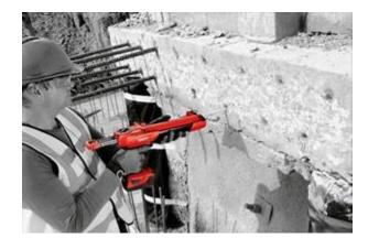
capacities, and smaller edge distances and spacings. Kacey pointed out that most documented failures using adhesive fasteners were due primarily to improper installation methods, most notably not cleaning the hole prior to installing the adhesive.
