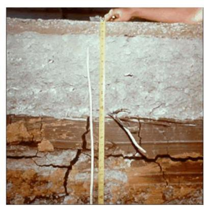
Basically, the last three cause the pavement to bend into a downward curvature at the edge of the pavement, thus making the transverse design a soil-structure interaction problem. All four are made more severe by the action of vegetation growing at the edge of the pavement and extracting moisture from beneath the pavement.
