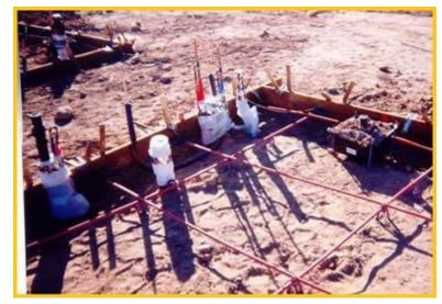
layout, and inspecting the plumbing and electrical work. He discussed methods of repairing plumbing and electrical lines after concrete placement. He also listed specific items to check proper to concrete placement.
