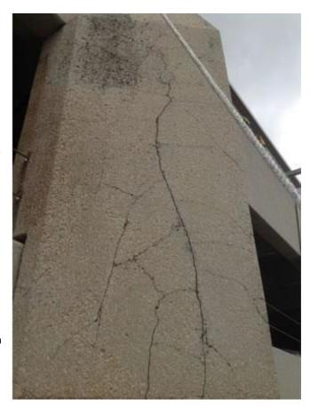
of the cracking on existing precast concrete columns consists of up-close field observations, non-destructive testing, material sampling, inspection openings, petrographic studies, structural analysis, and reporting.
