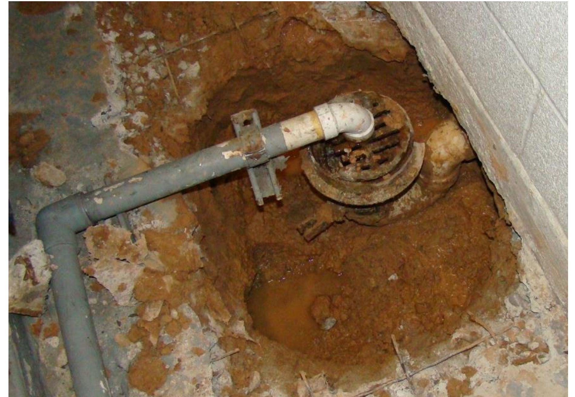
Water intrusion beneath the slab
