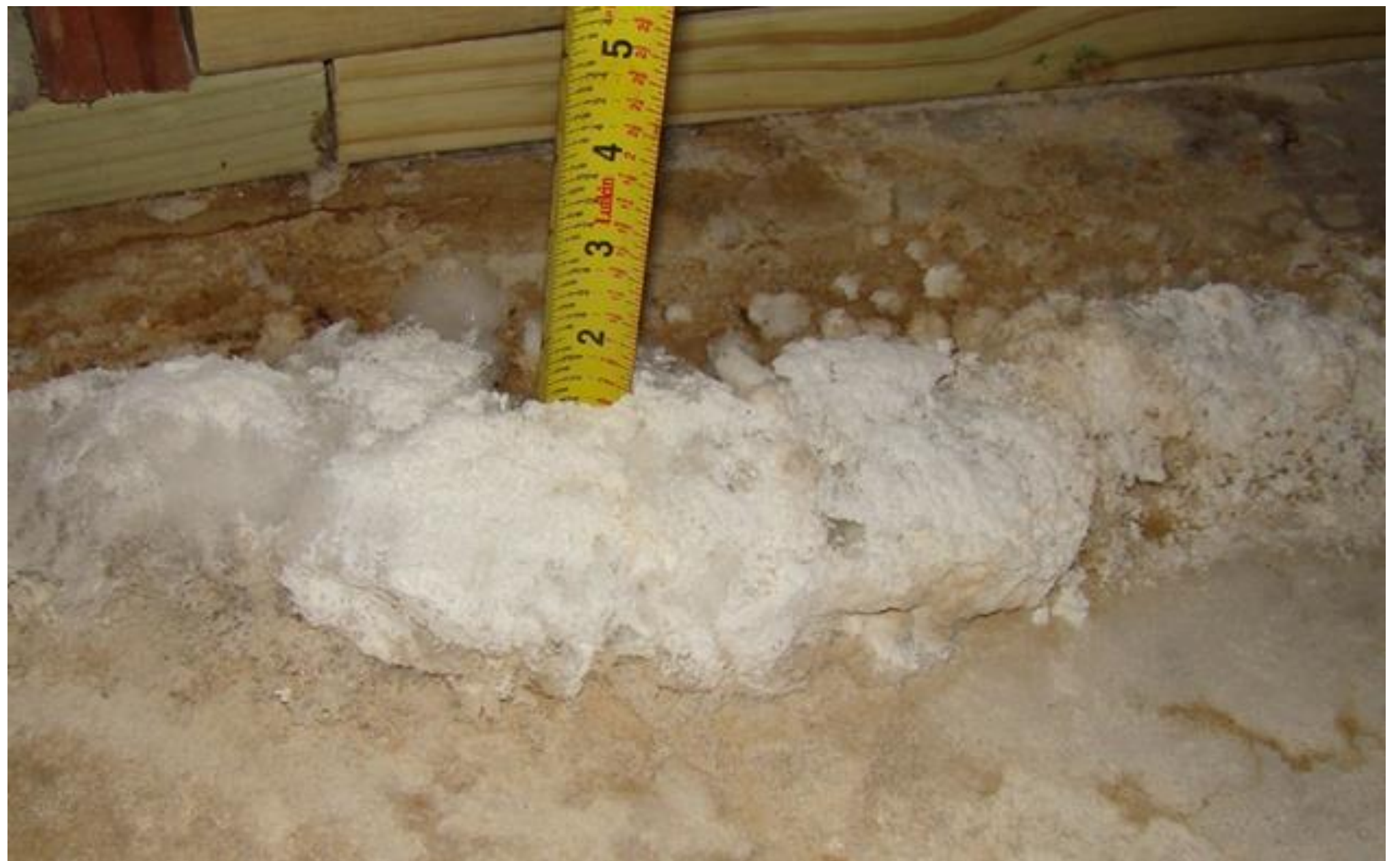
Efflorescence crystals due to moisture in slab
