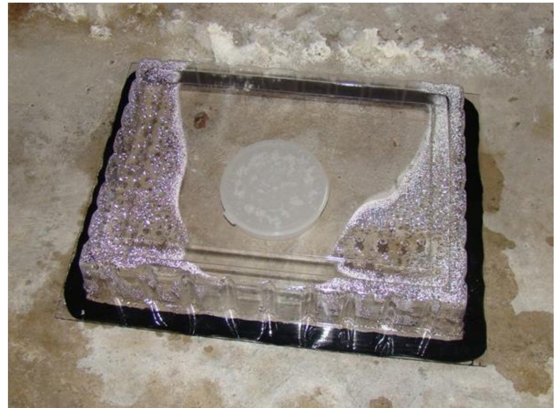
Condensation inside MVER dome
