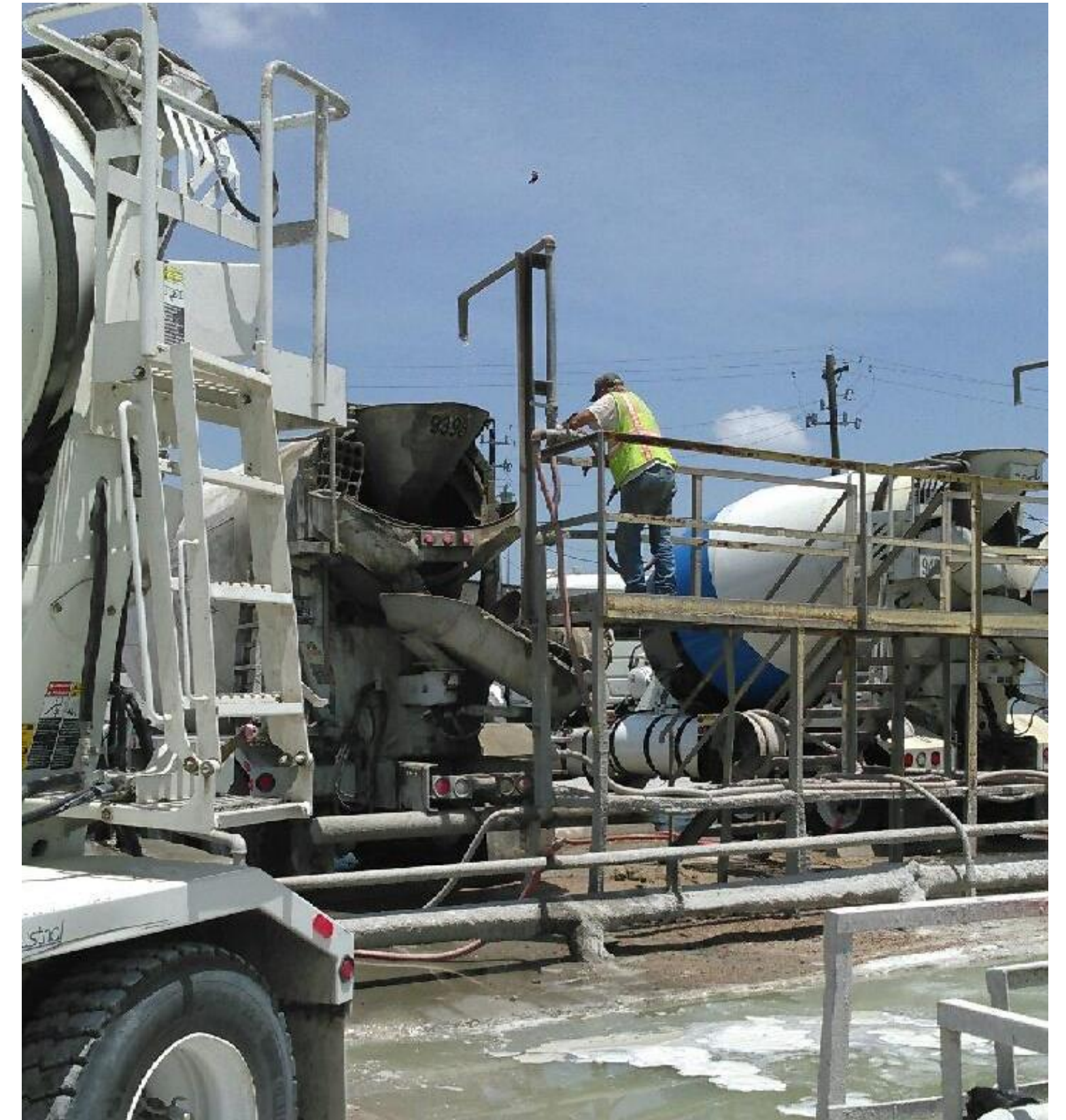
Adding 30 gallons at the slump stand
