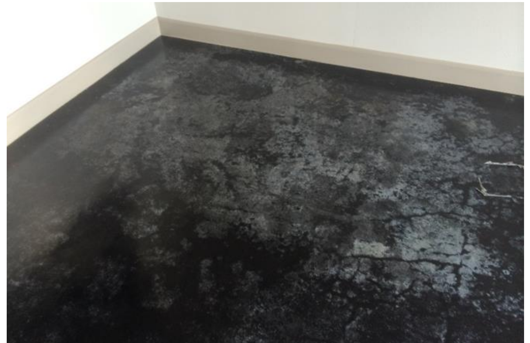
Efflorescence accumulated on slab
