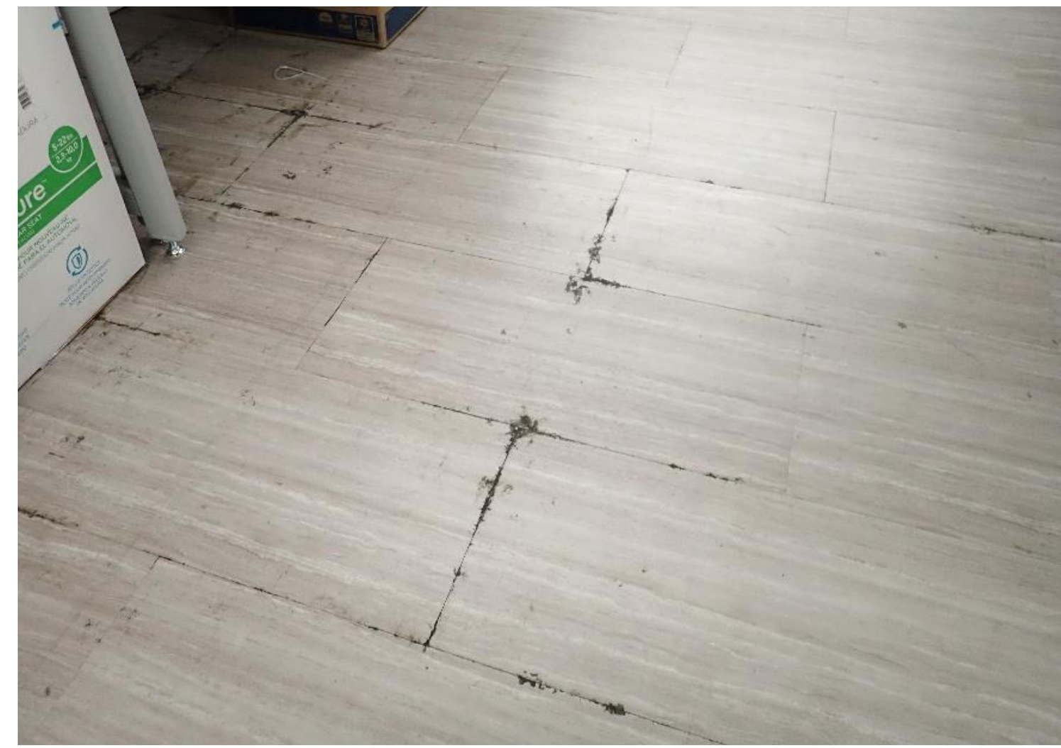
Adhesive bleeding through joints
