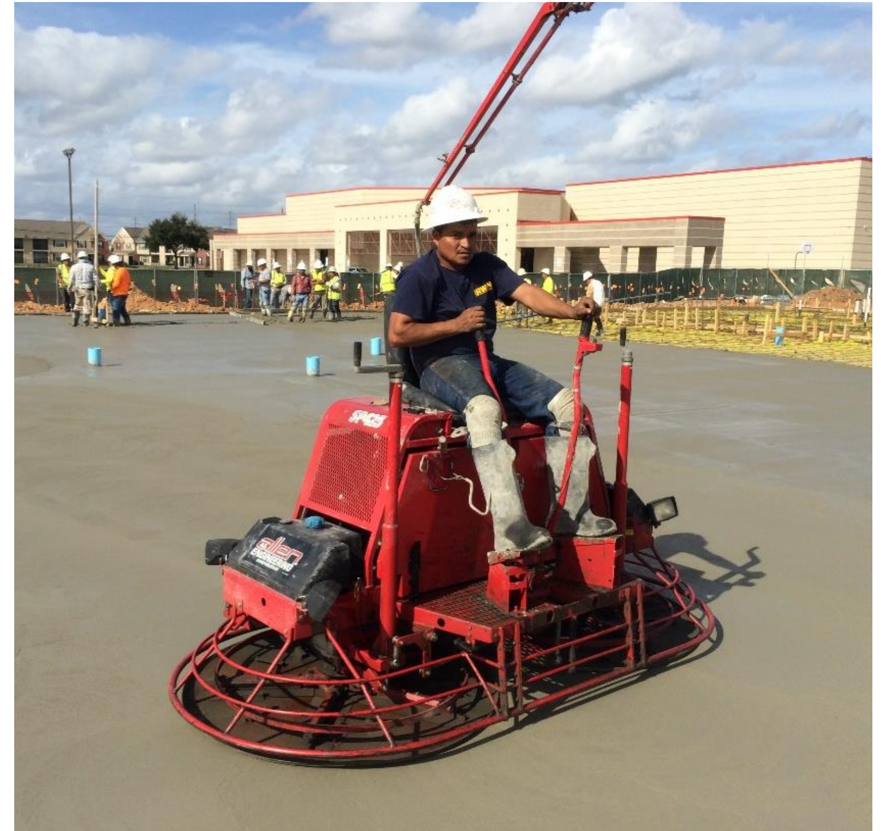
Trowel machine with pan floats
