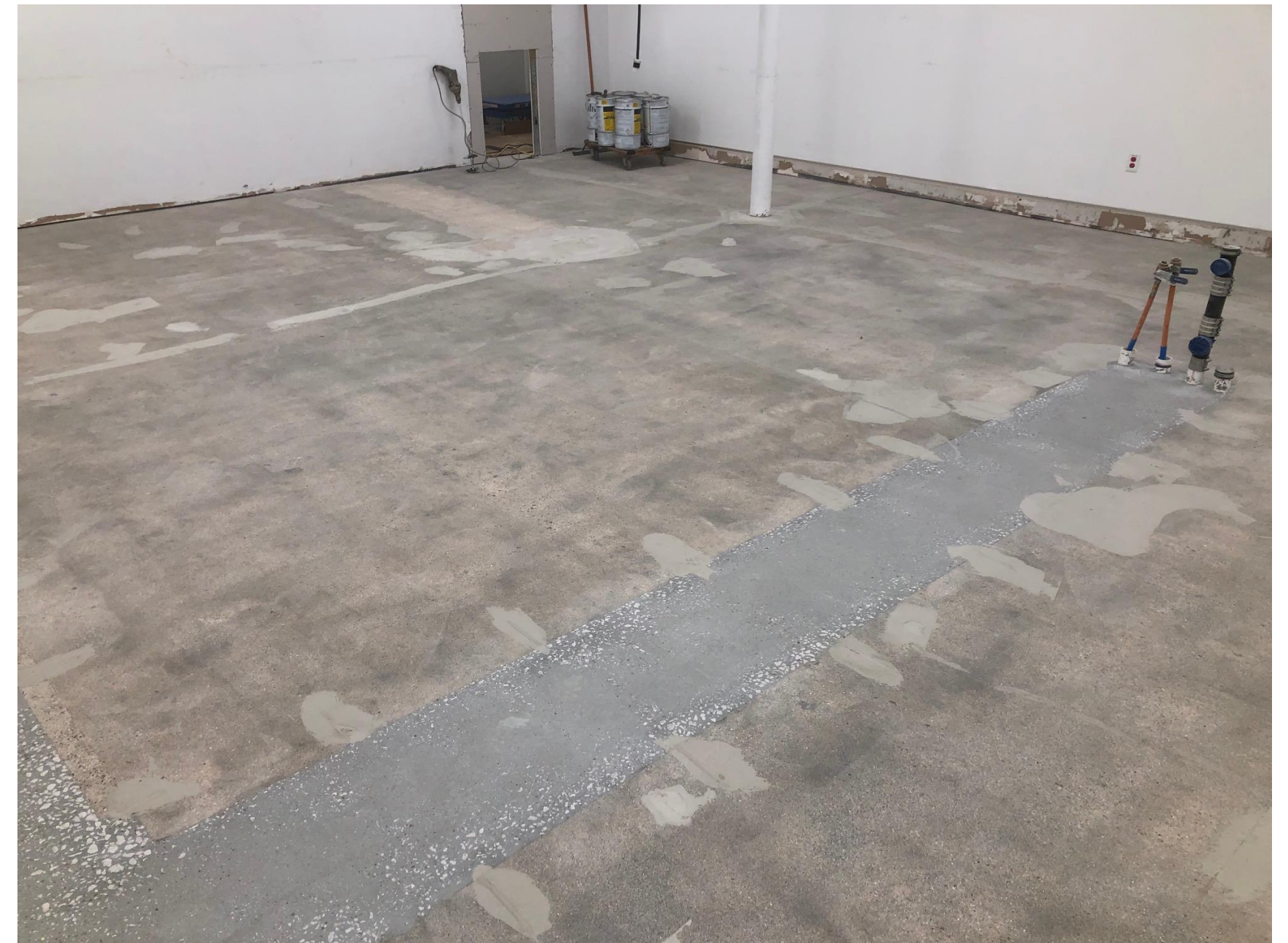
Concrete surface preparation
