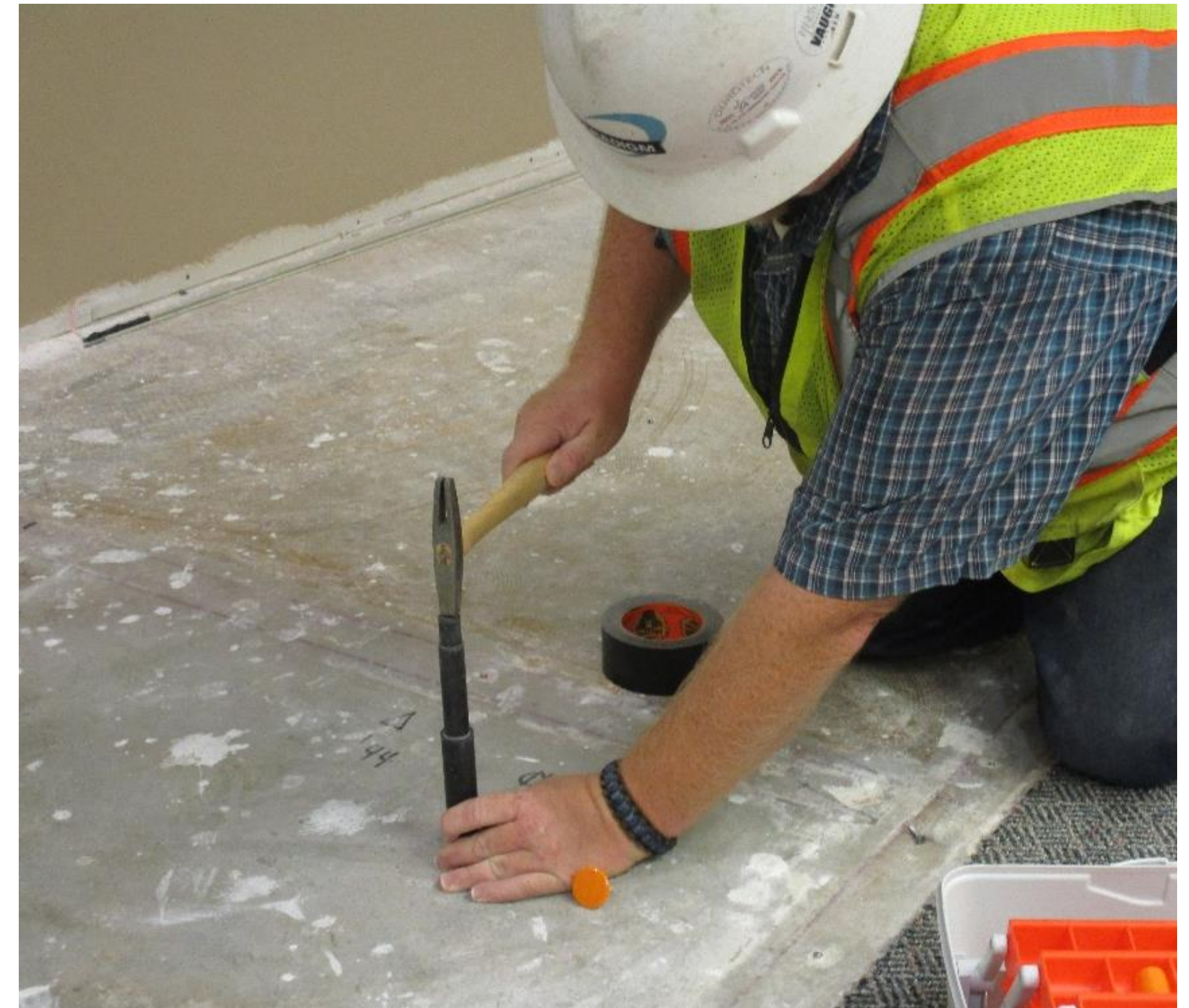
Installation of RH probes
