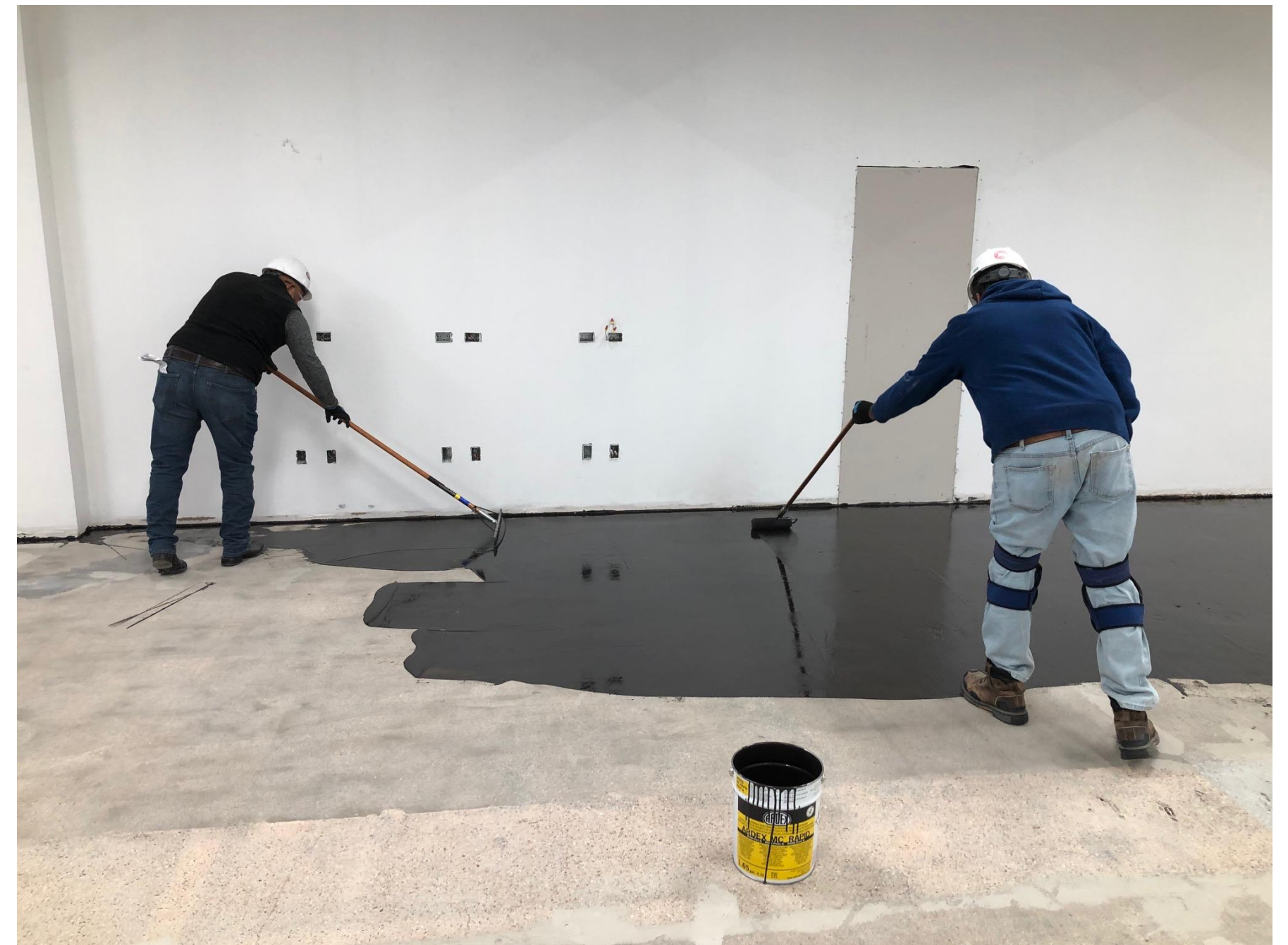
Application of moisture control system
