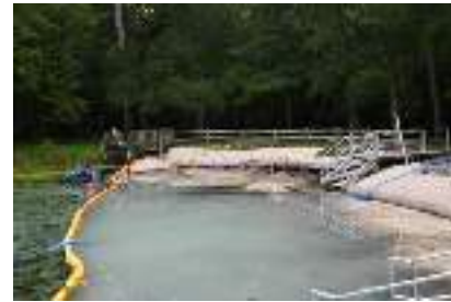
Fill SOX with organic media (blow-in compost, topsoil and dredge spoils)
