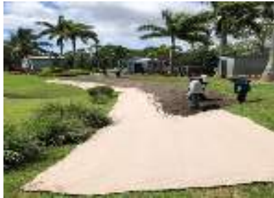
Fill SOX System with organic media (blow-in compost, topsoil, or dredge spoils).
