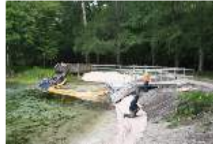
Layout SOX material & secure to Patented anchoring system.
