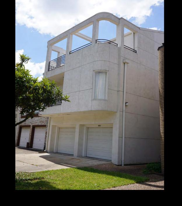
Maximizing space over 25' bldg. setback line: floor cantilevered 4' to add living space. Had to use 2x12's cantilevered out and going back twice as long inside garage to cross beam
