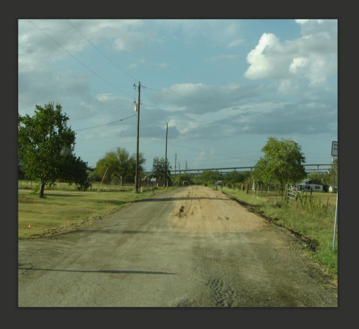
Earthlok injected the highlighted portion of the road. The remaining area was untreated.
