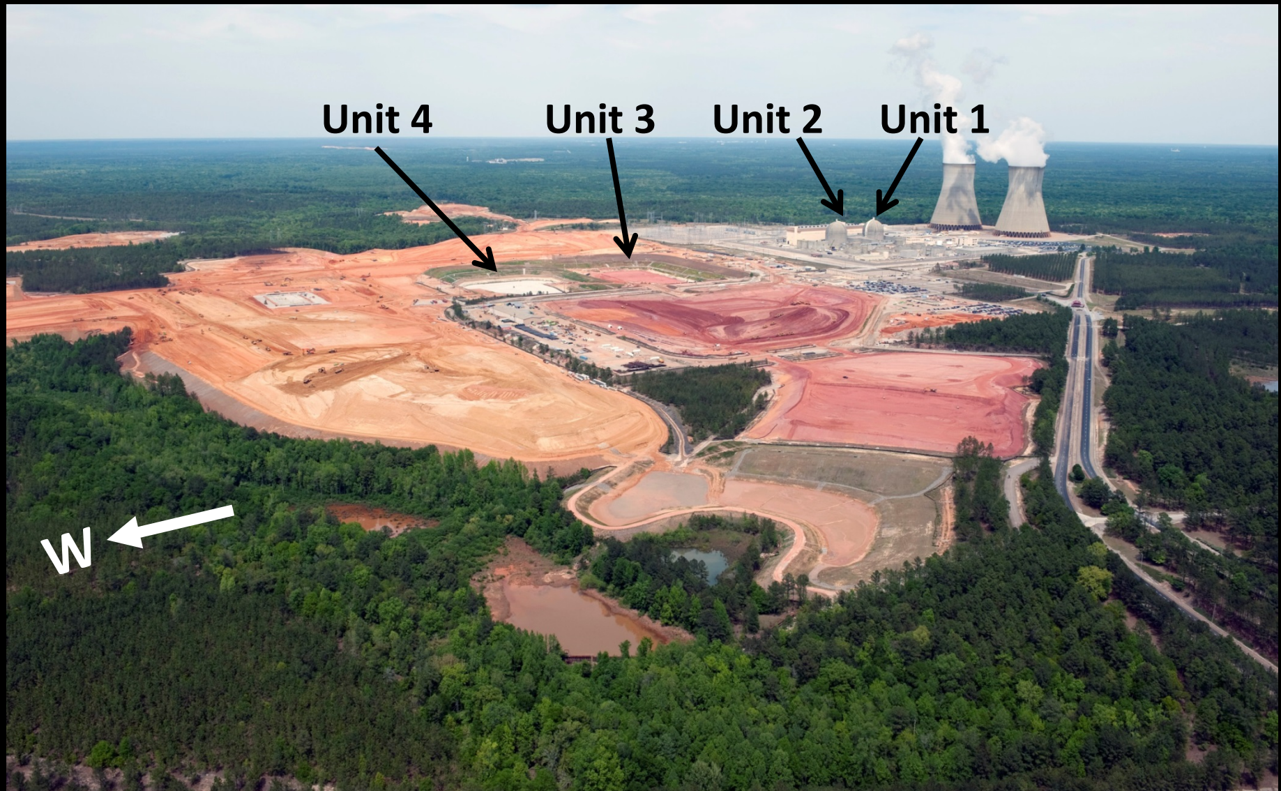
Plant Vogtle Units 3 and 4 foundation excavation, with water vapor rising from cooling towers in background. April, 2010.
