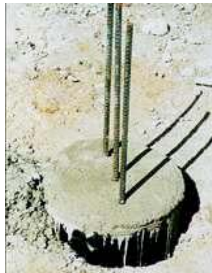
Forms around the upper 2 feet of piers eliminate flaring
