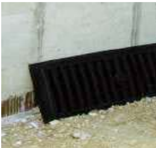
Example of a high-density polyethylene (HDPE) Soil Retainer manufactured of materials that are not adversely affected by moisture.
