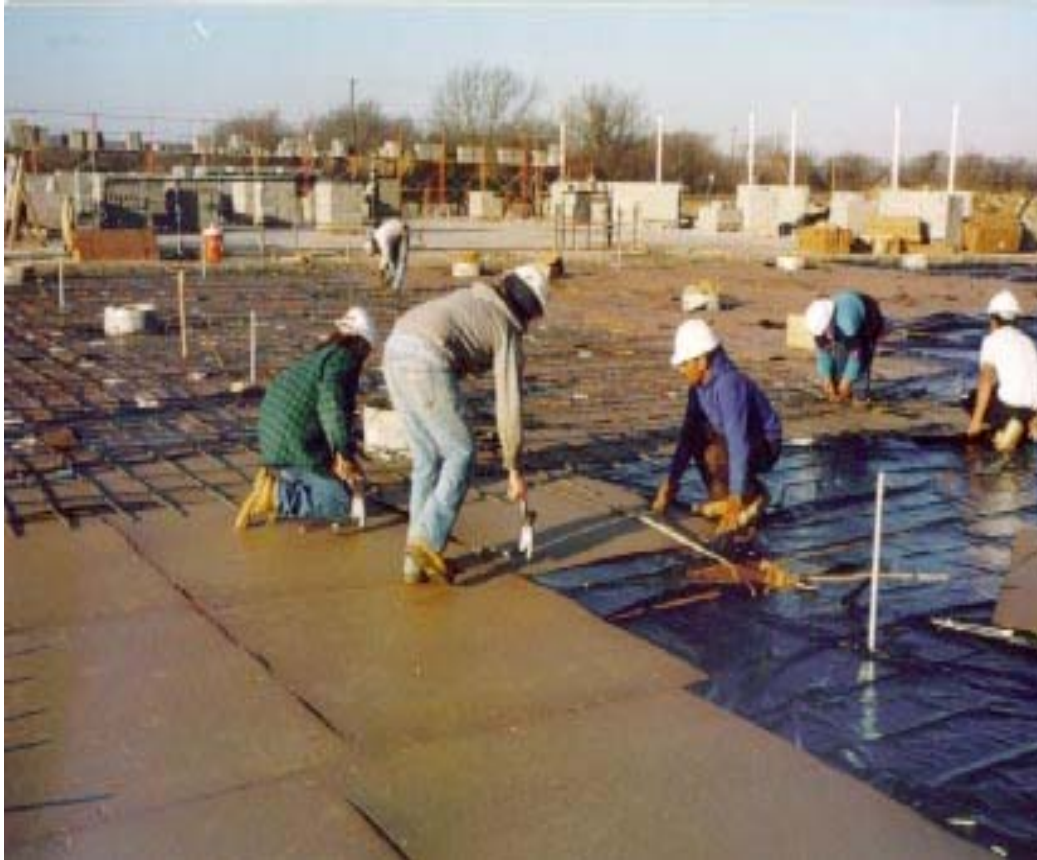
Protective fiberboard sheets being placed over Carton Forms
