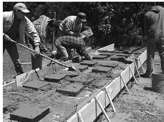
Placing concrete over boxes
