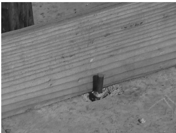
Slab indicators showing the “heaving” of the soil and therefore the failure of the boxes
