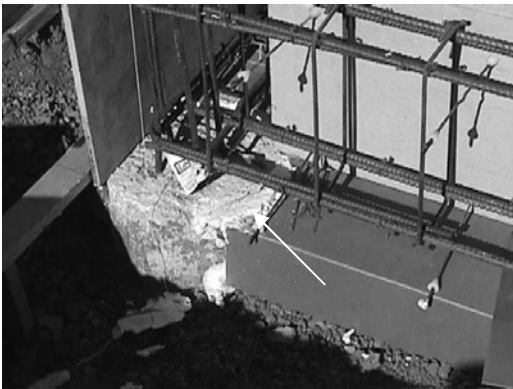
Expandable Foam used to fill gaps
