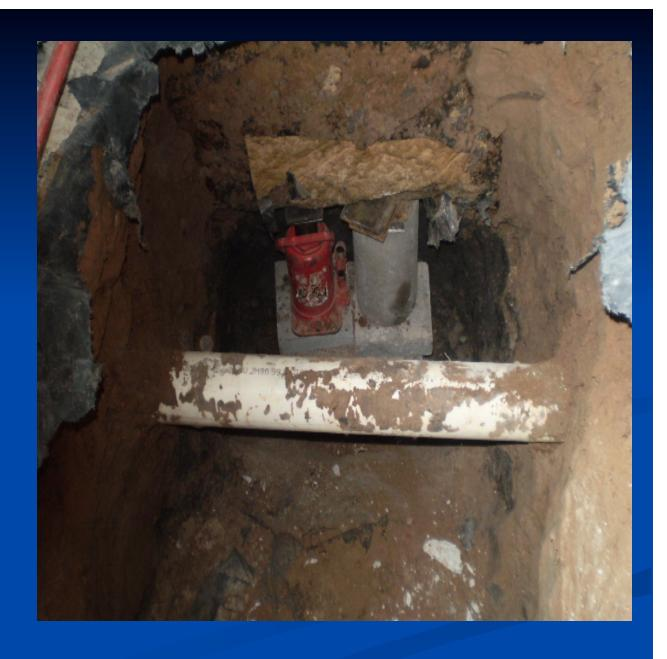
Lifting structure using hydraulic jacks
