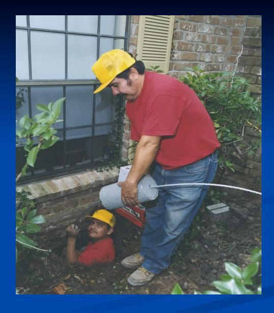
Driving concrete segmental piles using a hydraulic ram
