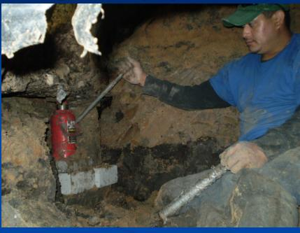
The weight of the structure is used to create the reactive force that allows the pile segments to be driven into the soil.
