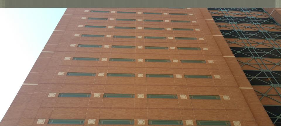
Hide joints with brick details. Put joints on inside corners.
